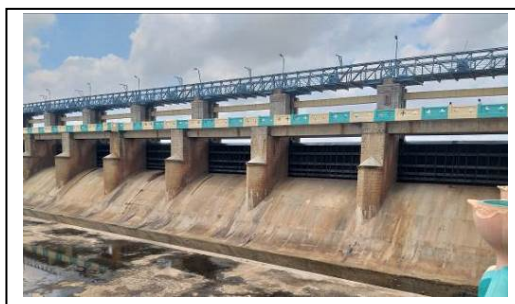
Renovated medium irrigation facility
