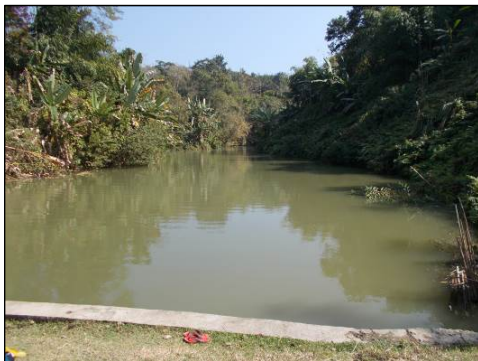
Check dam constructed
