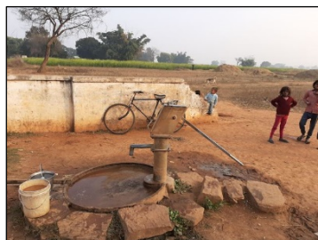
Water facility Pukhradh village, Mirzapur district
