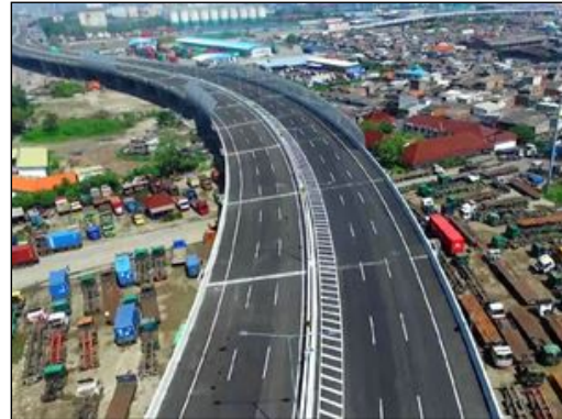
Tanjung Priok Access Road
