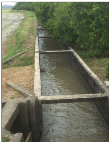
Photo 1: Irrigation Canal Facilities Constructed by This Project (Pampanga Province)
