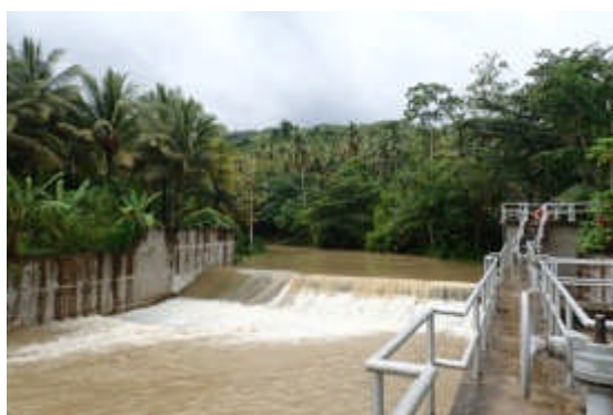
Photo 1: Water Supply and Sanitation Sector Small-scale Dam (Cebu, Visayas Area)
