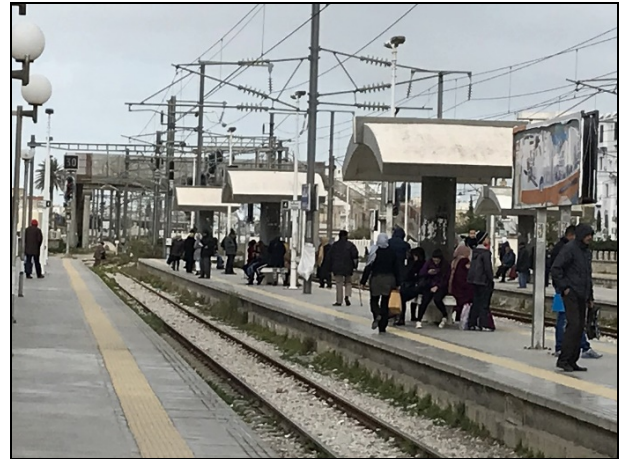
Haman Lif Station in target railway in the project
