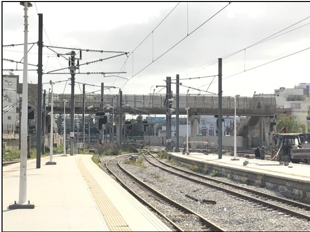
Carthage Bridge constructed by the project, a view from Tunis Station
