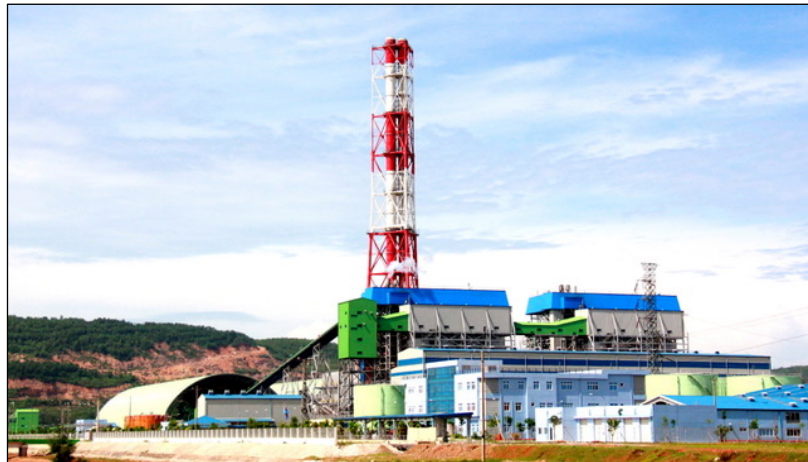
Nghi Son 1 Coal-fired Thermal Power Plant
