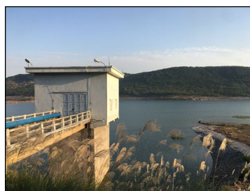
Ash Disposal Pond
