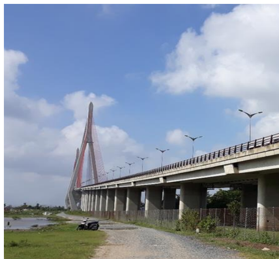
Can Tho Bridge
