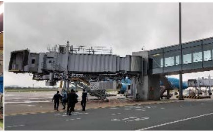
Passenger Boarding Bridge
