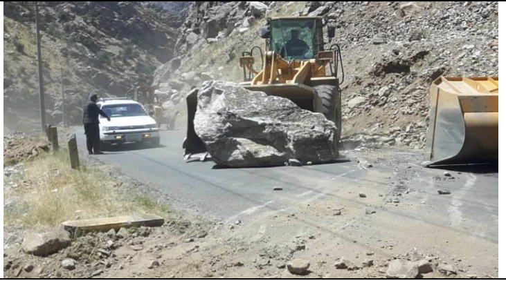
Routine maintenance work is ongoing at road site
