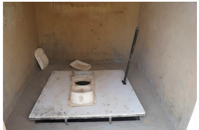
The pilot composting toilet in Barkoundouba village
