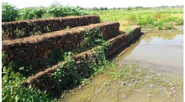
A reservoir in good condition in Bourdi 2, Tahoua region
