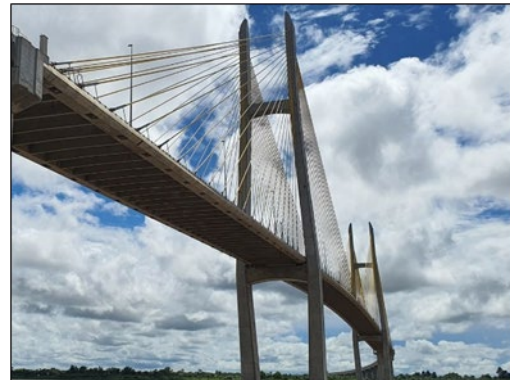
Neak Loeung Bridge
