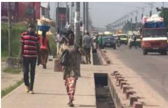
sidewalk, side ditch, road-curb
