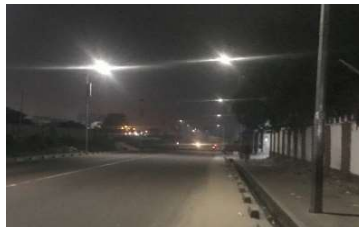
Streetlights at night
