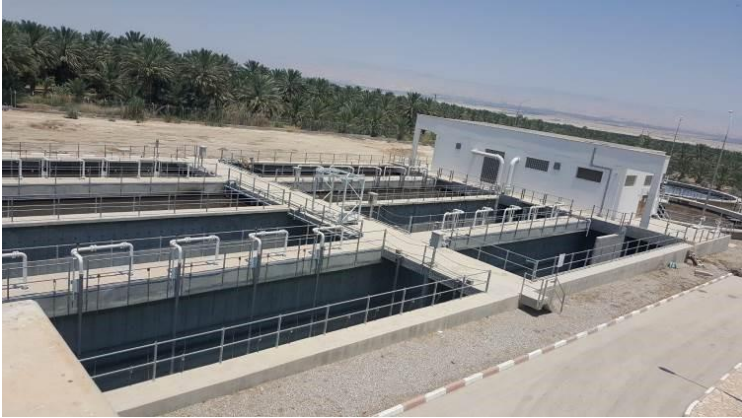
Well maintained facility by the staff trained by the Project
