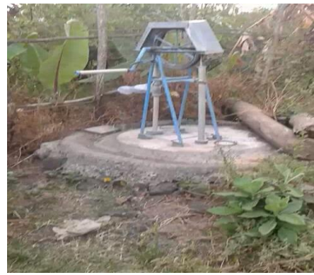
RP installed after the project in Meskan woreda. It was purchased with the fund from micro-finance.
