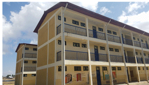
Secondary school constructed by this project
