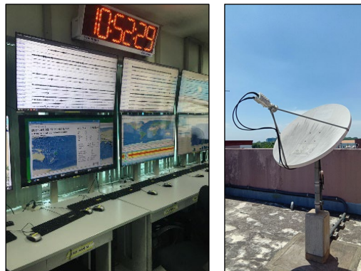
Equipment maintained by this project (PHIVOLCS headquarters monitors, IPSTAR satellite communication equipment)
