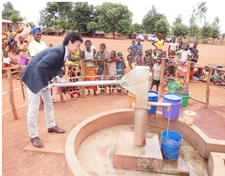
Local community can access to safe water through water points constructed under the project
