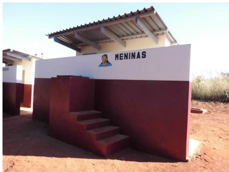
Sanitation in primary schools is improved through school latrines constructed under the project
