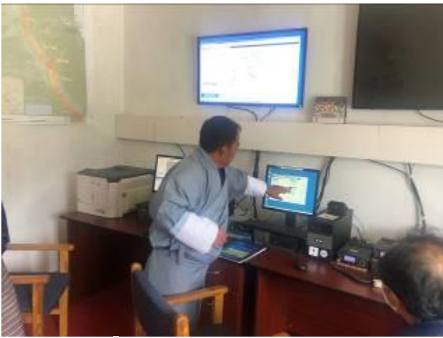
24/7 Manned Control Room at Kurjey in the Chamkharchhu Basin.
