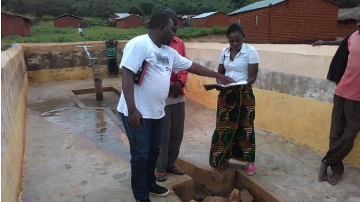
Molosiyo No. 2 Water Point in Mchinji, one of the boreholes constructed by the project. WPC has benefitted from the O&M training during the project.
