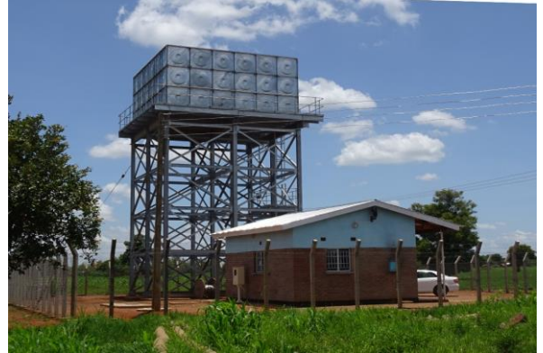
Water tank at Santhe market centre in Kasungu constructed by the project
