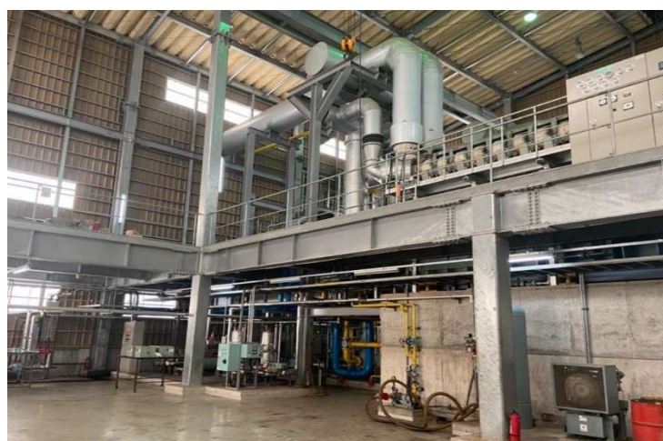
Interior view of the powerhouse building
