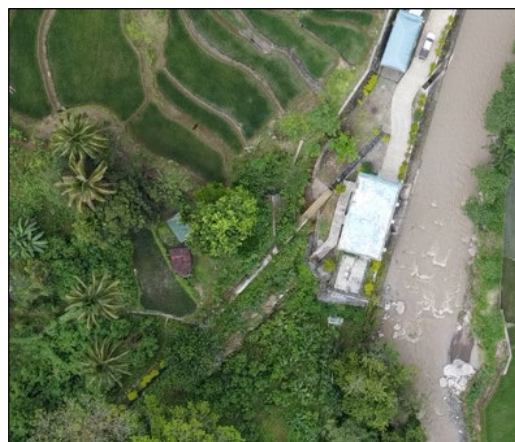
Constructed Likud Mini-Hydro Power Plant
