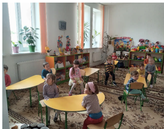
Photo 7: Learning room where pellet boiler heating equipment is installed (Mateuti Kindergarten)
