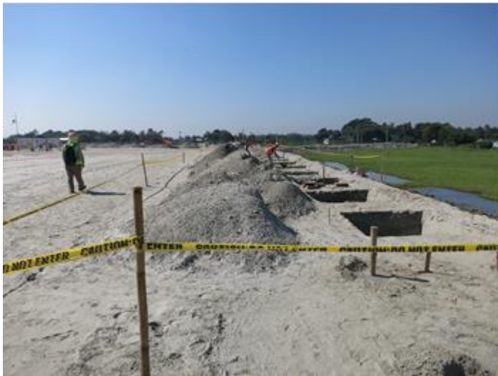
Construction site in the Bangladesh Special EZ
