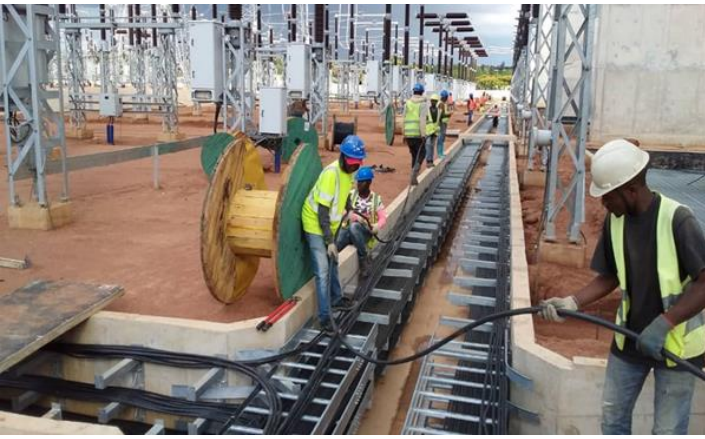
Cable laying at the site of Shinyanga Backbone Transmission Investment Project
