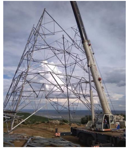
Tower erection at the site of Kenya-Tanzania Power Interconnection Project
