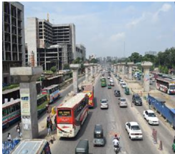
BRT Line 3 construction of piers near Shahjalal International Airport
