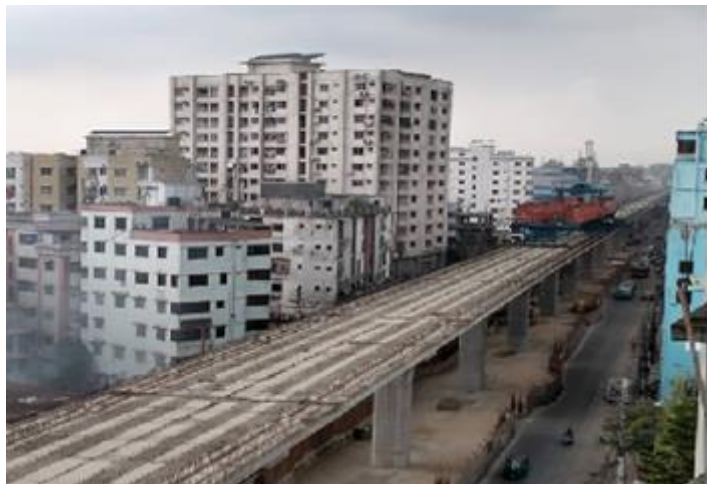
MRT Line 6 construction of elevated section near Kazipara Mirpur
