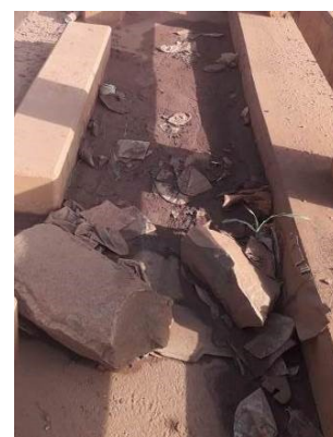
Wastes left on the sidewalk
