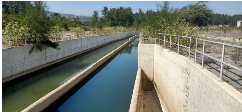
Photo 1: Irrigation facility developed by this project (Main canal) (1)
