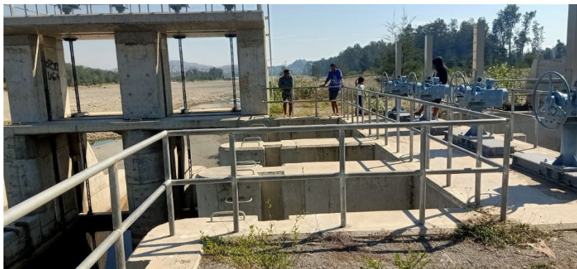
Photo 3: Irrigation facility developed by this project (Weir)
