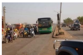
Condition of the road before implementation of the project 18
