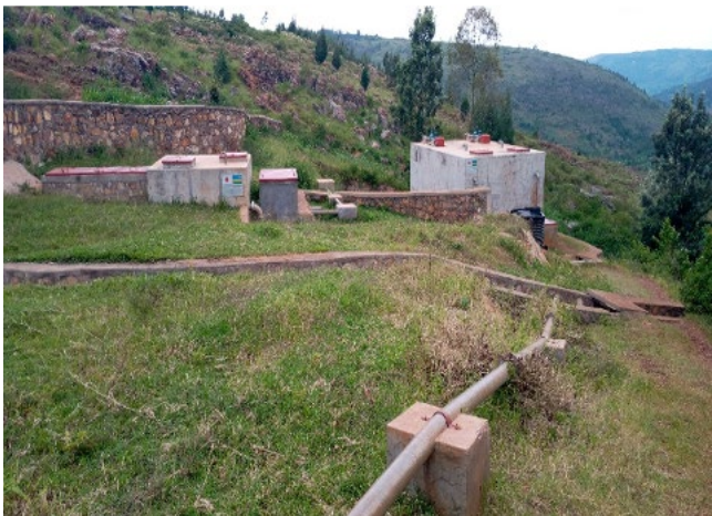
Spring intake facility (left), receiving tank (right), transmission pipeline (foreground) (Rukira Sector, Ngoma District (Rukira East))
