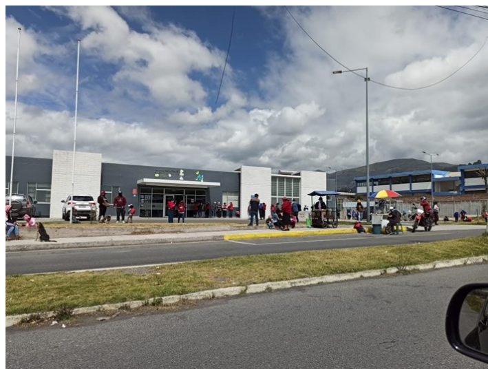
Carpi health center constructed under this project
