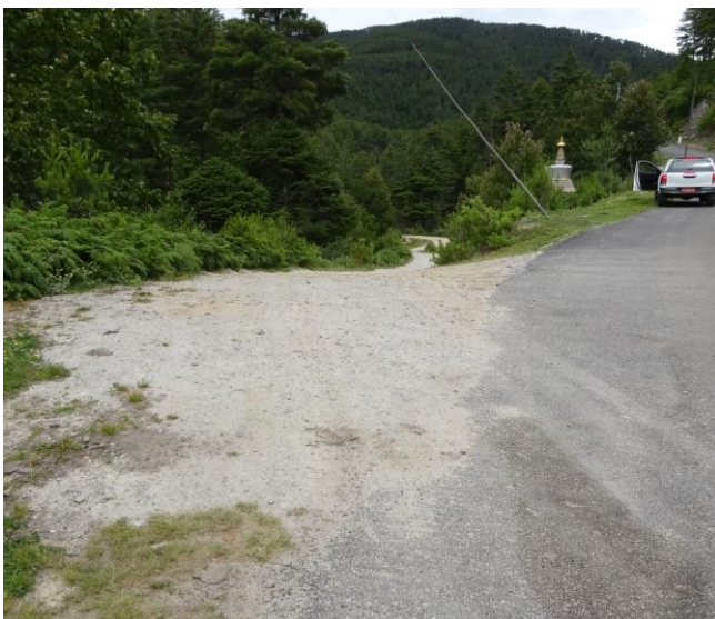
Farm Road constructed by using the procured equipment in Bumthang District connecting national highway, making easy access to the public facilities for the people of Chungphel Village.
