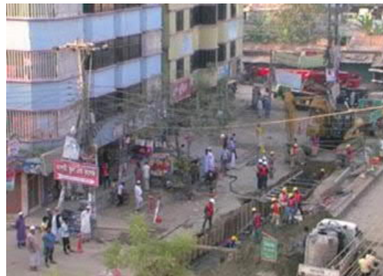
Photo 3. Work to lay distribution pipes (photo from JICA's project documents)
