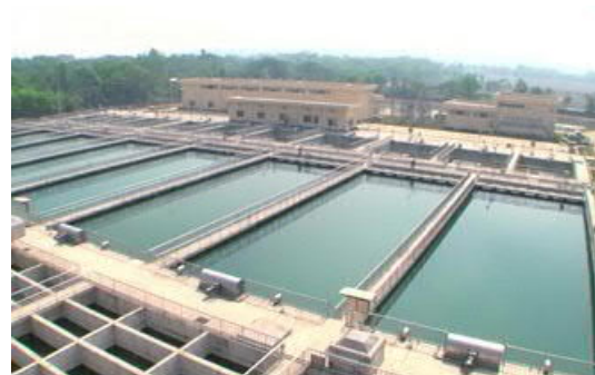
Photo 1. Karnaphuri water treatment plant constructed by the Project (a photo from JICA's project documents)
