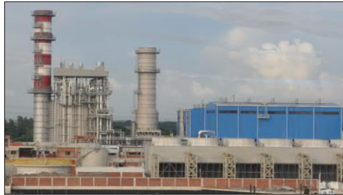
New Haripur Power Plant
