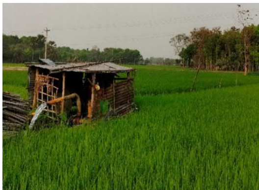
Electric Power Pump for Irrigation (Jessor PBS, Khuluna Division)
