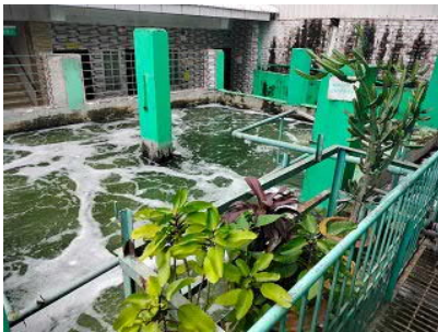
Photo 2 Wastewater treatment facility
