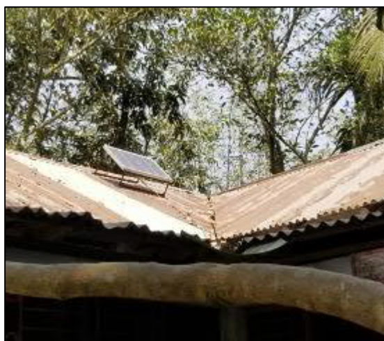
Installed Solar Panel for SHS
