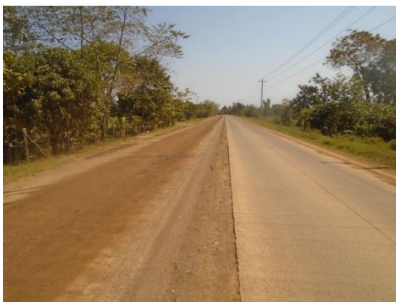
Unpaved part of Section 3
