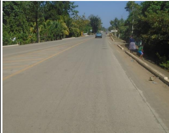
National Highway No.7 East (Section 4)
