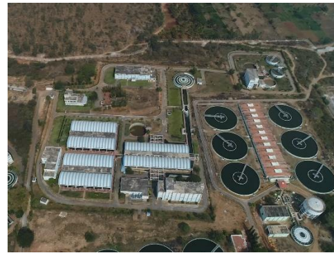
A bird's-eye view of the T.K. Halli water treatment plant (Photo courtesy: Executing Agency)
