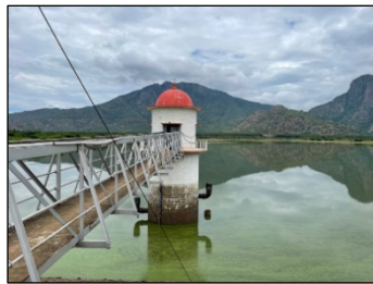
Water Intake Facility (Dindigul)
