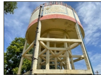
Water Storage Facility (Devakottai)
