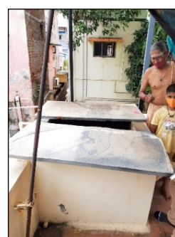
Rooftop Water Storage Tank
