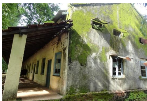
Hostel at SFTI Shahapur (Before renovation)
