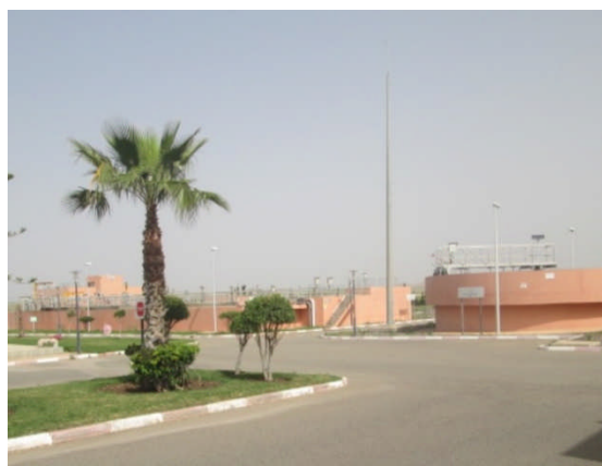
Photo 2: Overall view of the sewage treatment facility, constructed with OCP funds (Ben Guerir City)
