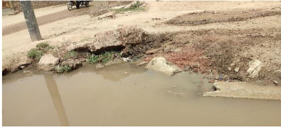
Figure 9. Damaged Side Protection at Tulwala Distributary
