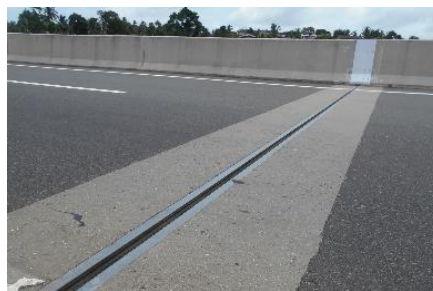
Expansion joint in other sections
