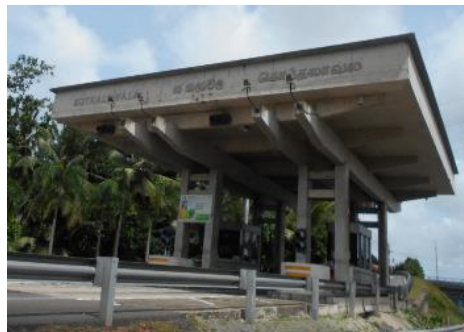
Additionally constructed Kothalawala IC
