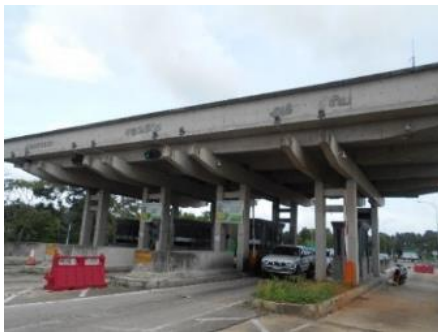
Additionally constructed Athrugiriya IC
