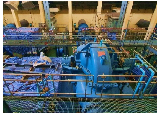
Raw water pump (left) and transmission pump (right) at Bangkhen WTP
