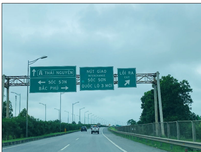
National Highway No. 3 constructed by the project
