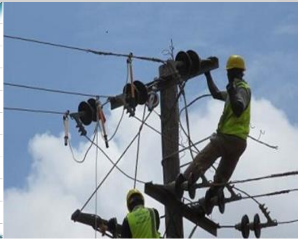
On-the-job-training (OJT) of maintaining distribution lines (Source: Terminal Evaluation Report p23)
