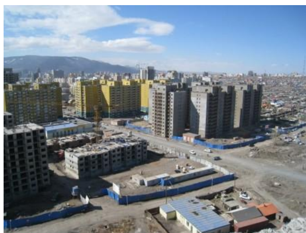
Results of an old apartment houses reconstruction project
